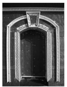
Plastic Components' **Casing Beads** create a termination point in many areas when applying exterior coating materials. They protect the coating with a straight, rustproof, high-impact resistant edge. Casing beads are versatile components that can be used on walls to create aesthetically shaped details and
