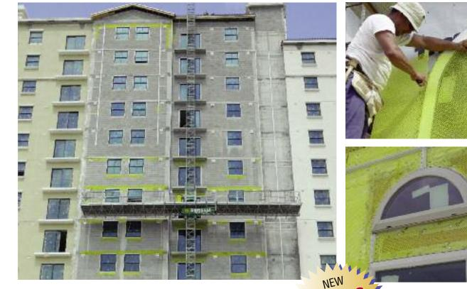
Plastic Components' Ultra-Lath Plus™ plastic lath is the labor-saving, non-rusting alternative to metal laths. It now
