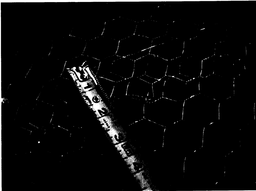
Photograph No. 2 - Typical 1" Woven Wire lath overlap and wire ties
