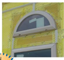
Plastic Components' **Ultra-Lath Plus®** plastic lath is the labor-saving, non-rusting alternative to metal laths. *It MEETS ASTM and comes backed with asphalt-impregnated paper for superior moisture control.*
