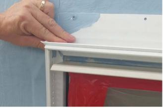
One-piece **CONTINUOUS INSULATION TRIMS** for hard coat combine a weeped foam TRAC<sup>TM</sup> with a corner bead for improving job quality in foam, with 3/4" or 7/8" stucco finishes
