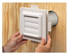
1 Cut hole in substrate with a 4-1/2" hole saw. Insert vent tube into opening.
