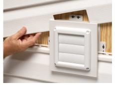
**3** Install siding. Overhang on vent flange hides cut ends of siding.
