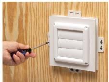
**2** Use screws to mount dryer vent to substrate through flanges.
