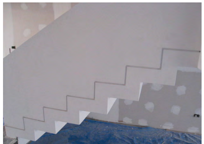
Aesthetic Drywall Reveal and 90° Angle Reveal Intersection in staircase
