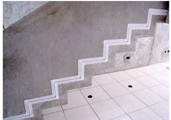
Aesthetic Drywall Reveal and 90° Angle Reveal Intersection in staircase
